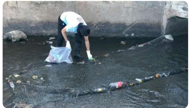
Pilot containment nets in a drainage channel, Maputo
